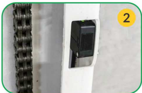
2. Photoelectric detection, to detect existing car or something else under to ensure safety (Fig. 02).
